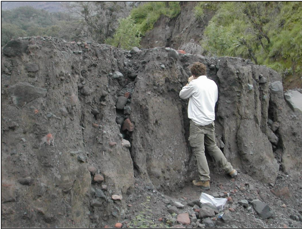
Figure A5: Site 4 with a blackened tree stump.
